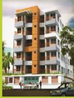
DISHARI MOMTAZ VILLA 25/12 Rupnagor Residential Area
